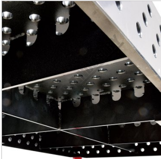
Strengthened by Welded Webbing
