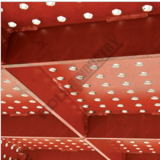
Strengthened by Welded Webbing
